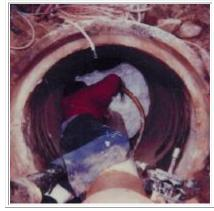
A technician filling the final 10 feet of the pipe. Note how the Tripolymer completely fills the pipe interior, as the technician slowly pulls the applicator hose toward him. In this picture it is necessary to point out that Tripolymer does not expand upon installation - the complete fill is achieved by a pressure application method.
