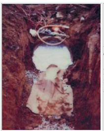
A job completed - This particular job took 33 days to complete and consumed 43,100 cubic feet of Tripolymer 105-Tank Media Foam. In this picture, the final section has been foamed and awaits only a minor touch up before it can be sealed. Our patented mixing gun can be seen atop the pipe.
